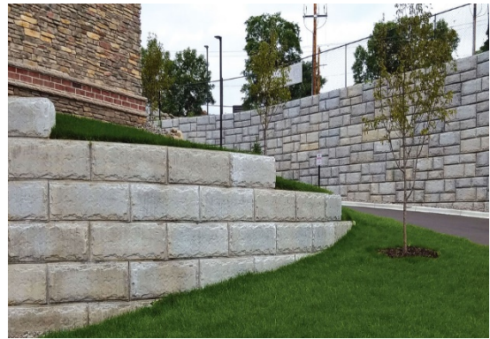
"Big Block" precast modular block walls Photo Credit: Versa-Lok
