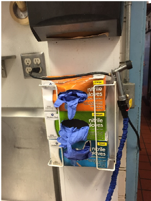
Devices at wet areas.
