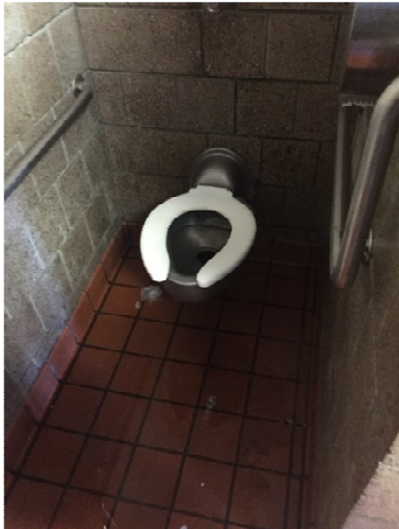
Men's public restroom water closet.
