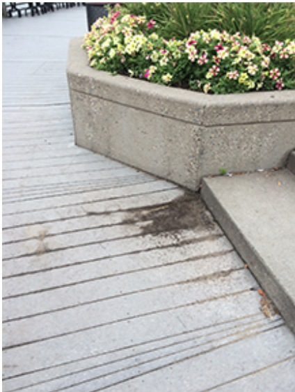
Warping composite deck.
