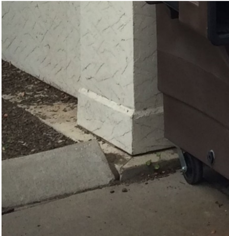
Mortar joint at stucco base.
