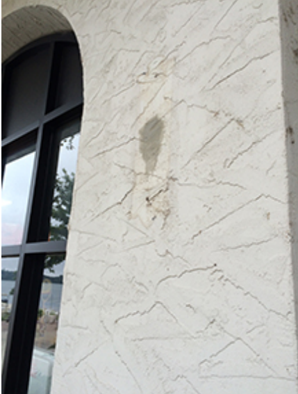
Area at removed fixtures.
