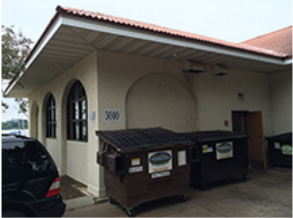
Grease hoods at exterior wall.
