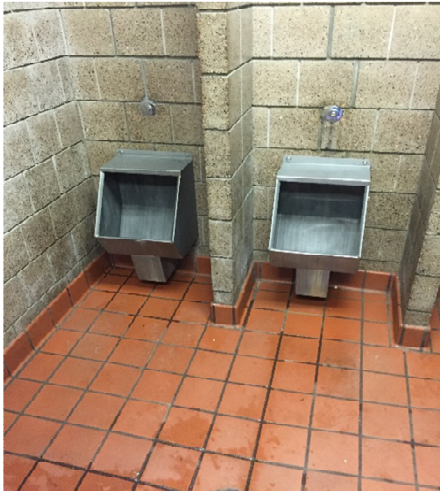
Men's public restroom urinals.
