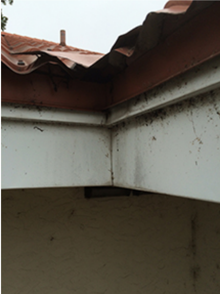
Roof tile at eave.
