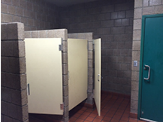
Women's restroom stalls.
